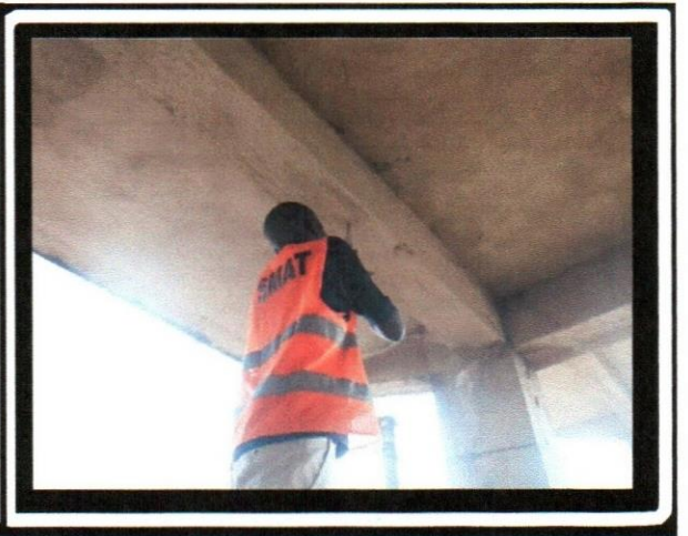
Rebound Hammer test to find the insitu concrete strength/ Surface hardness.
