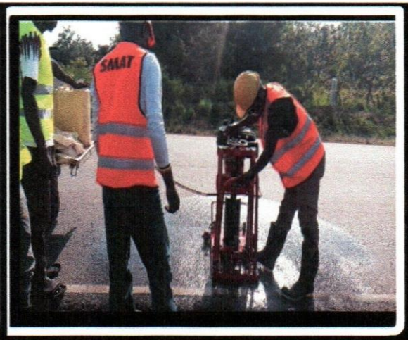
In-situ Asphalt concrete coring to determine the Voids content.
